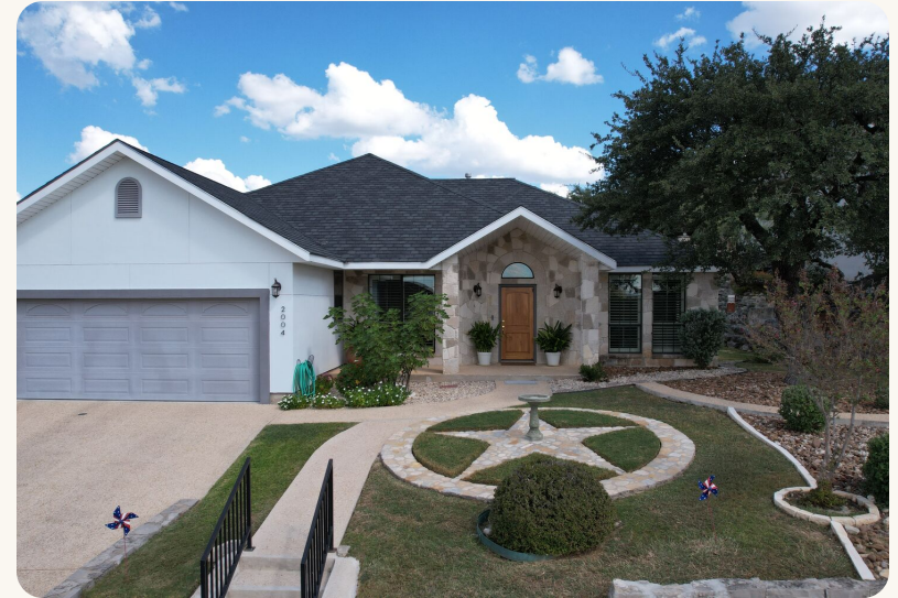
The front of the house — stone and stucco, a two-car garage, and a landscaped front lawn the association maintains.
